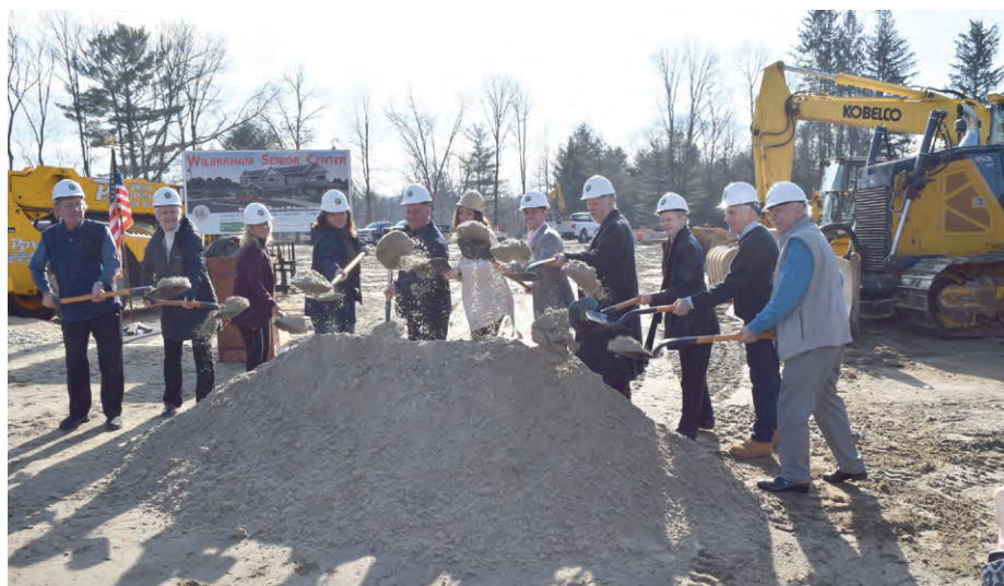
Ground was broken on the new Wilbraham senior center on Feb. 10.
