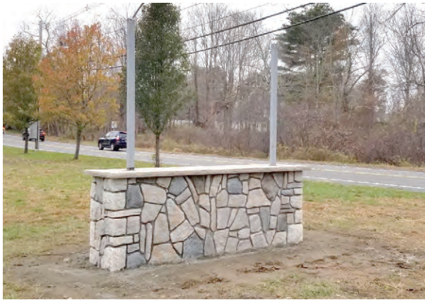
Although what it will say is still not obvious, the base for the signage as one enters the property is a work of masonry art!
