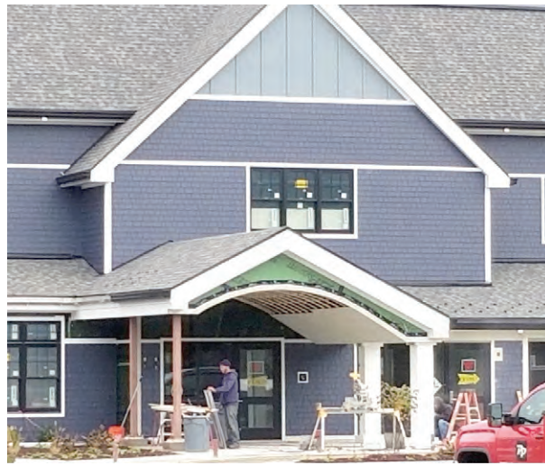
Our main entrance is taking shape! The area is covered by a portico to make access easier in inclement weather.
