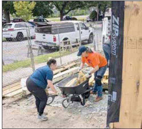
Appleton moving concrete at Dwight St.
