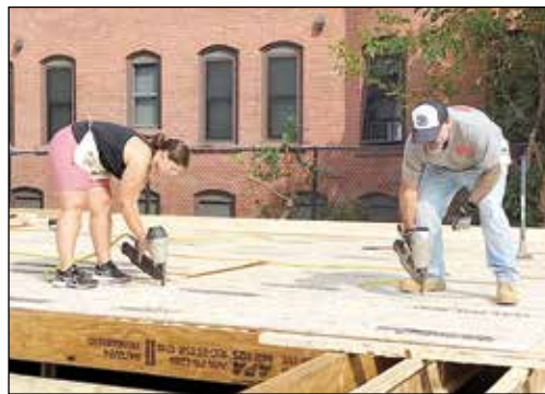
Springdale nailing in base floor at Dwight St.
