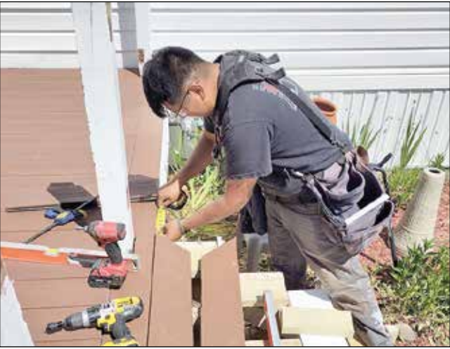
ABOVE: Edgar measuring deck: Edgar Herrera of Greater Springfield Habitat for Humanity's construction crew works on the new deck.
