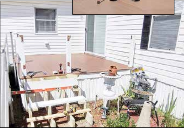
Wayne's new deck while it's under construction.
