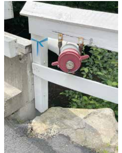
The fire department uses this device to pump water from the Scantic River at the bridge on Rock-A-Dundee Road.
