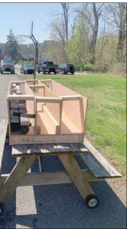
Photo and caption courtesy of Hampden Fire Department The Hampden Fire Department completed a prop for training, sharing these photos on Facebook: "Our day crew recently constructed this prop for training for the department. This prop simulates a hose bed on an apparatus and will allow our members to practice pulling a hose line from a fire apparatus."
