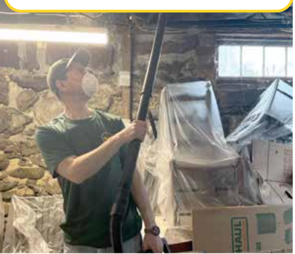
The basement ceilings also got some sprucing up.
