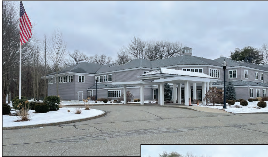
Turley photos by Dalton Zbierski. The Mental Health Association is moving its headquarters to the former MassMutual building on Memorial Drive.
