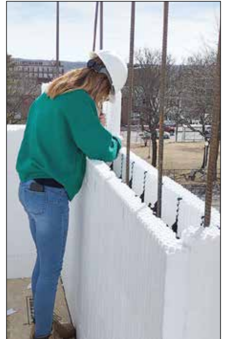
Dean student working with rebar at Chestnut.
